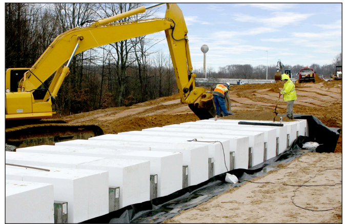
EPS Geofoam Protection
